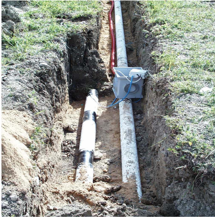
Pic.4 - Installation of relay for defect insertion
