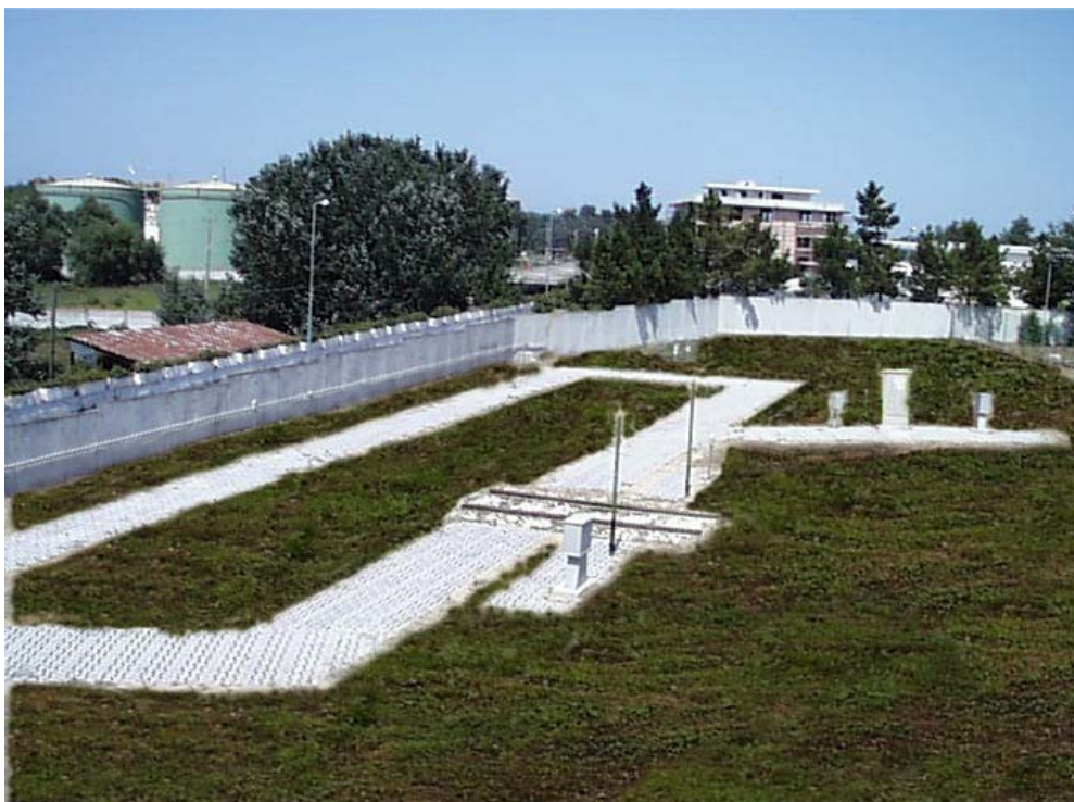
Pic.2 - Panoramic Wiew of the cathodic protection testing field "DX" side
