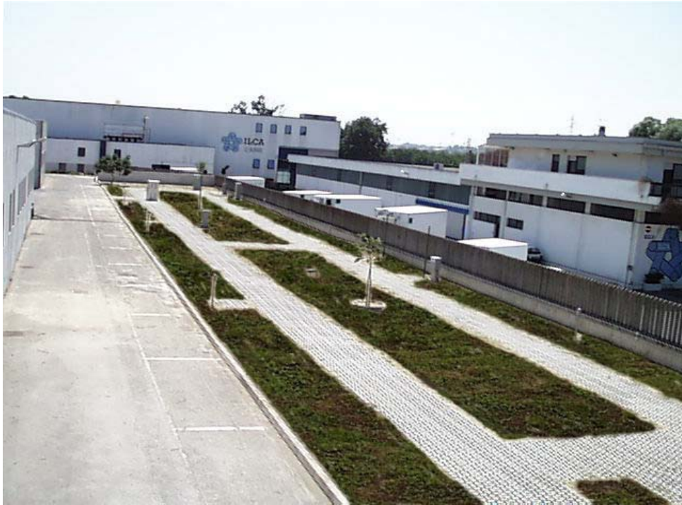
Pic.1 - Panoramic Wiew of the cathodic protection testing field "SX" side
